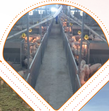
The pig farm construction and assistance project in Zhaojiaping Town, Xing County, Shanxi Province
