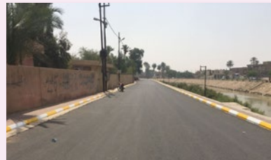
Before and after road renovation in Musharrah, Iraq
