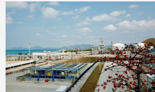
Hainan branch's green factory
